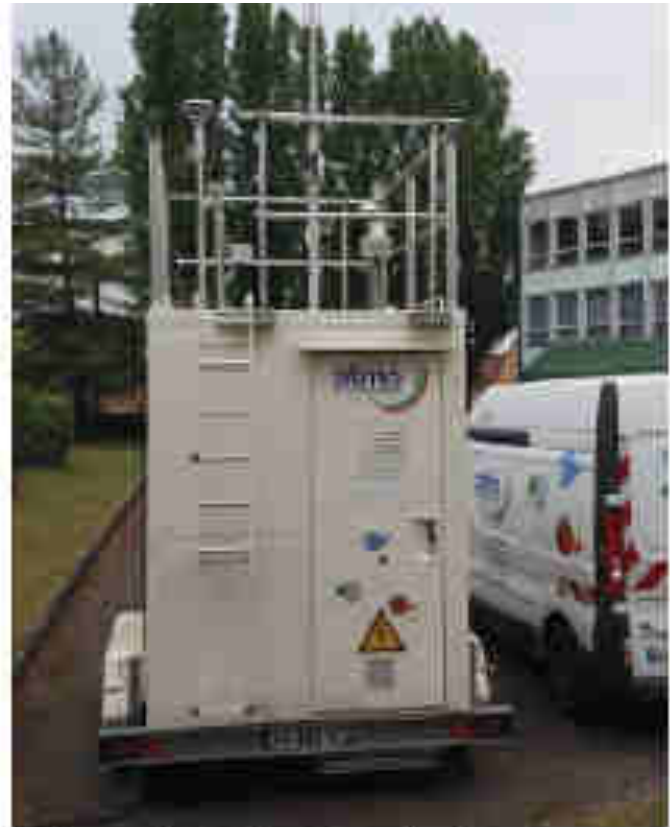
Station mobile à Marly © Atmo Hauts-de-France
